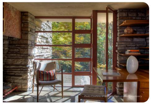
The Western Pennsylvania Conservancy uses *Starphire Ultra-Clear®* glass to replace window and door glass at Fallingwater. The work is done on a routine basis at the historic house, usually in conjunction with steel conservation.
